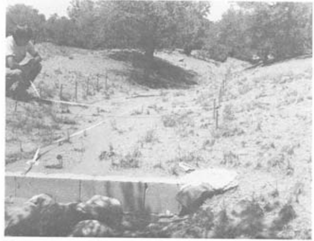
FIG. 17. Photograph of Big Sweat Dam, basin of Arroyo de los Frijoles, near Santa Fe, N. Mex. The dam is shown in foreground; view is looking upstream at wedge of sediment deposited behind the dam. Vertical rods are steel pins used as permanent markers for resurveys.
