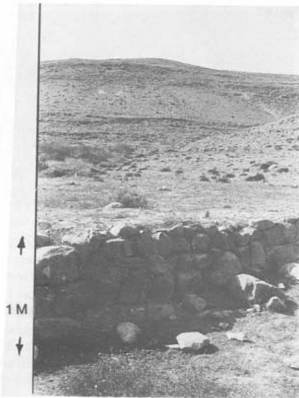
Fig. 1. Typical dam constructed nearly 2,000 years ago by the Nabatean people of the Negev Desert, Israel. The dams are typically about 1 m high, 50 m long, of rock blocks without mortar. View looking upstream across the deposited sediment. Photo by the author.
