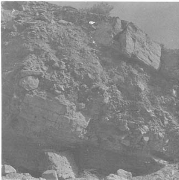
FIG. 7. View of coarse grained valley fill in the West Arroyo of the Loop at station 83+50.
