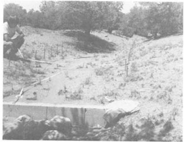
FIG. 17. Photograph of Big Sweat Dam, basin of Arroyo de los Frijoles, near Santa Fe, N. Mex. The dam is shown in foreground; view is looking upstream at wedge of sediment deposited behind the dam. Vertical rods are steel pins used as permanent markers for resurveys.
