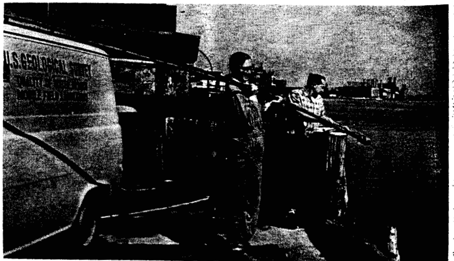
Installing a submersible pump to supply a continuous water sample to water quality monitor. At left is mobile laboratory used for special water quality investigations.
