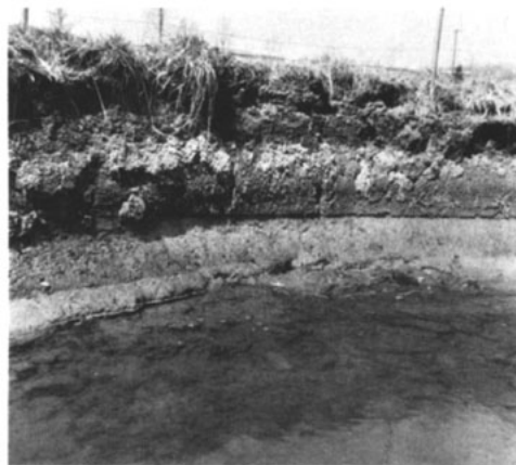
Figure 9. Stream bank which had been subject to ice crystal growth and loosening of surface layer. A moderate stream rise has removed this prepared material in lower third of the bank leaving a fresh surface of silt and showing the main mechanism of bank retreat.
