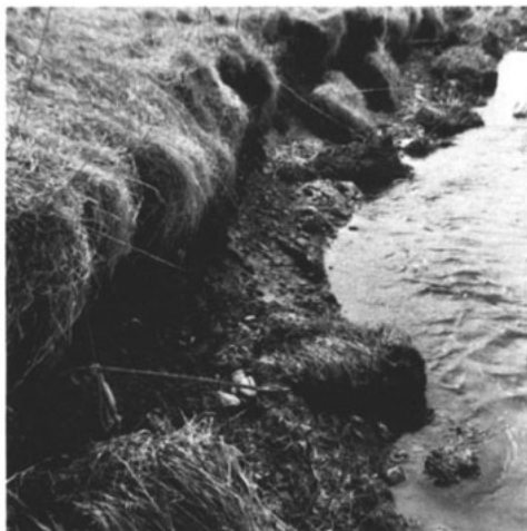
Figure 8. Closeup of retreating bank near section 44A-45 in 1971. Iron pin originally set well away from bank has been exposed by bank retreat and is now bent over into channel. Sod lumps undercut by bank retreat fall into channel.
