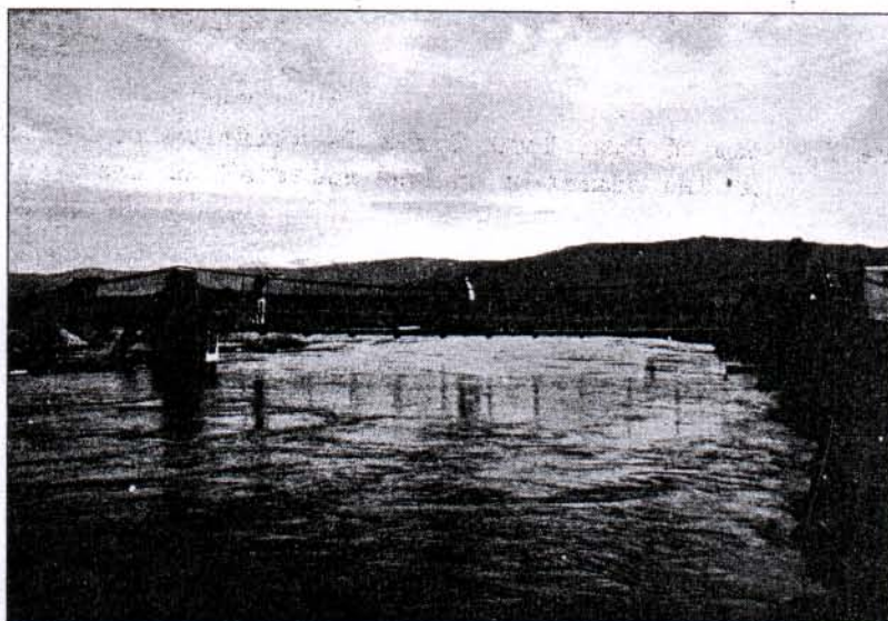
B. View downstream at suspension bridge; flow is relatively high.
