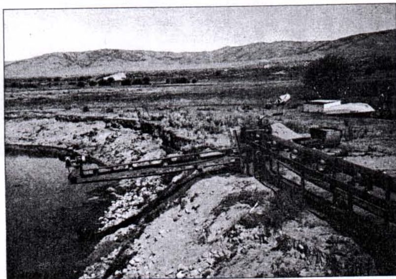
DOWNSTREAM BELT DELIVERS SEDIMENT TO RIVER BELT AND THUS TO RIVER
